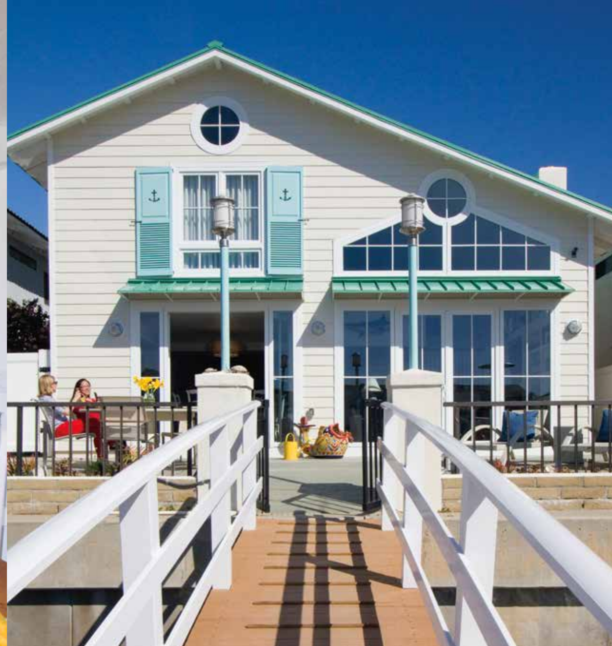
The rear of the house faces an inlet where Coronado Cays' residents dock their boats.
