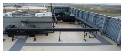
Completed tower roof, no coating was necessary
