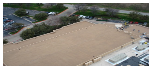
Finished upper roof area with aggregate
