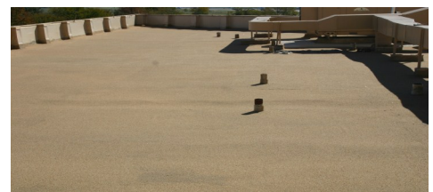
Finished roof area with aggregate installed
