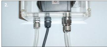
**2.** The reservoir/pump should be connected to the water-blocks and radiator in a loop. If you are using a second reservoir the outlet should connect to the bay reservoir pumps inlet.
