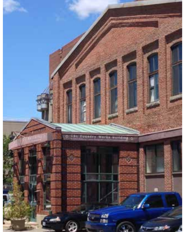
Historic facade with entry addition, facing Rogers Street
