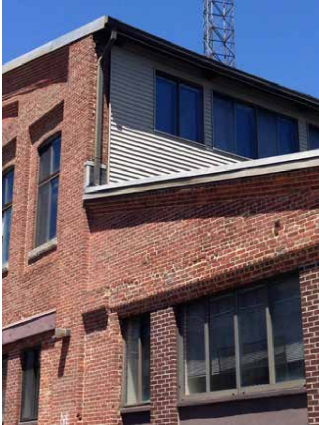
The wings of the buildings have clear heights up to 17 feet.
