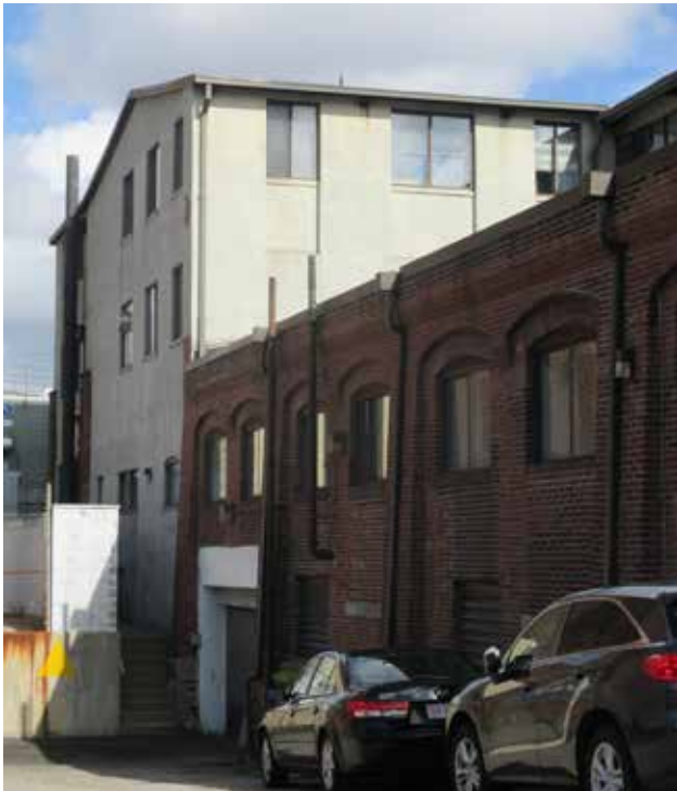
A driveway ramp leads to basement parking.
