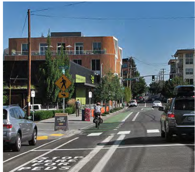
A continuous cycle track and improved streetscape can encourage more bicycle-oriented development, similar to the Williams Avenue corridor in Portland, OR.
