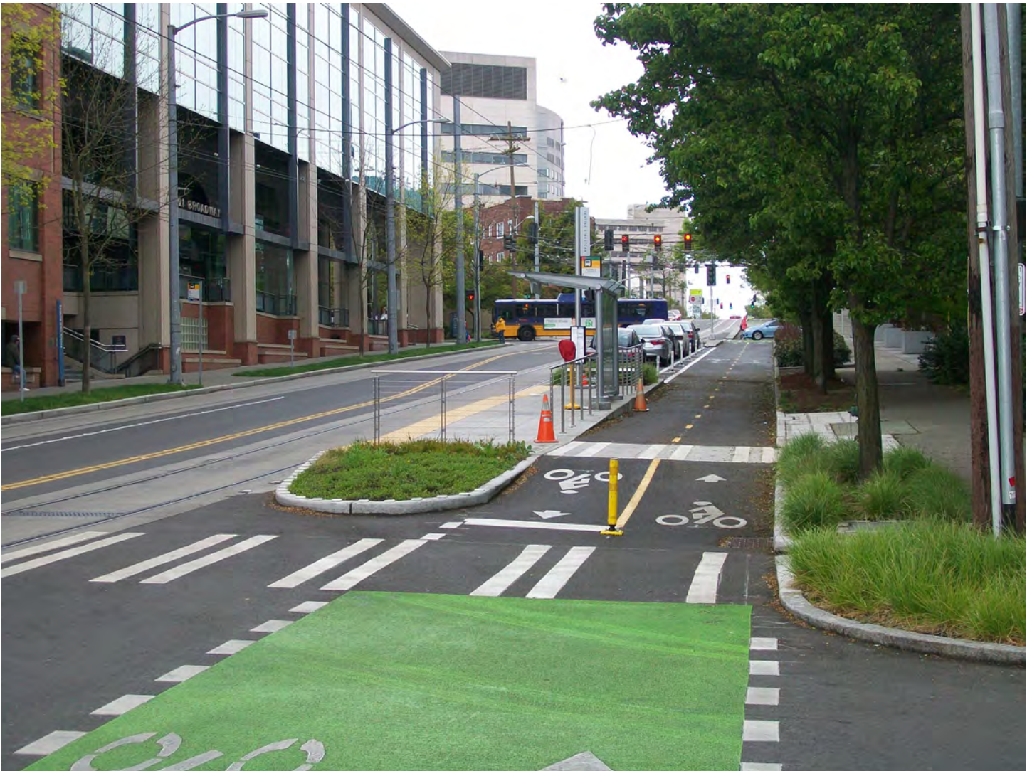
FIRST HILL CYCLE TRACK, BROADWAY, SEATTLE, WA
