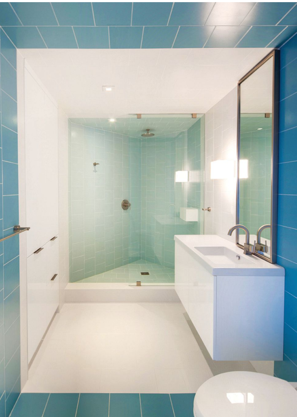
Imola Plain Series 8- x 8-inch tiles from Italy in three colors — azurro, aquamarine and white — were staggered vertically on the walls and floors of the children's bathroom.
