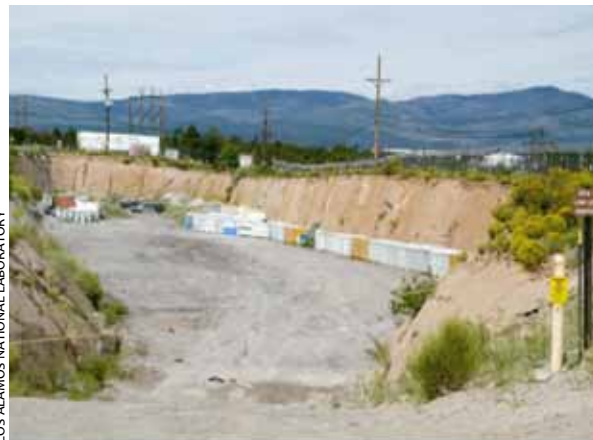
Until 1970, plutonium waste was dumped in unlined trenches at many DOE sites. It may never be cleaned up.
