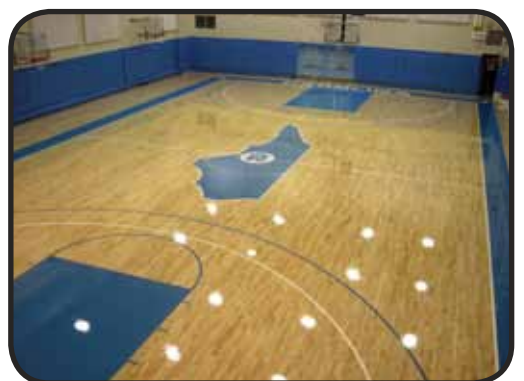
Robbins Springaire System University of North Carolina Installed by: Foster Specialty Flooring
