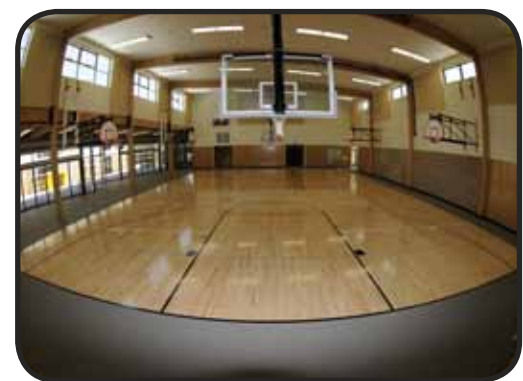
Robbins Bio-Cushion® Classic and Pulastic® Fusion System Trillium Creek Primary School Installed by: Brandsen Hardwood Floors
