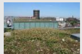
Office buildings in Basel. All new commercial buildings in Basel must be extensive green roofs which use local river terrace gravels and local wild flower seed mix to benefit invertebrates
