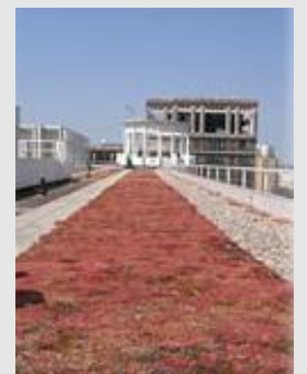
A sedum roof, Barking and Dagenham, London.
