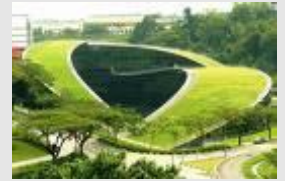
Organic green roof at the School of Art, Design and Media at Nanyang Technology University, Singapore.
