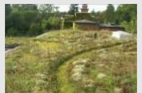
The modern extensive green roof system was born by accident. The first 6 storey concrete tenement blocks in Berlin in the late 19th century had bitumen covered roofs that became a fire hazard. These were covered with a layer of sand which would be colonised by self-established vegetation. roofs.
