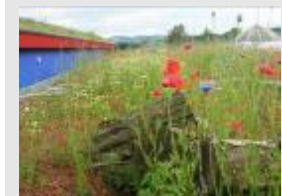
Extensive green roof using shallow, crushed brick substrate on a factory in Switzerland.
