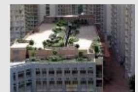
Intensive green roof in Hong Kong. There is an aim that green roofs will be retrofitted on existing Government buildings. Pilot schemes to install vertical green panels at lift towers and external walls will also be carried out in public housing estates.
