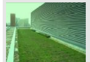
Extensive green roof at First Street, Manchester, both during and after installation.
