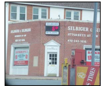
The coldest temperature I saw on the Silbiger Building was -3°F early one morning.
