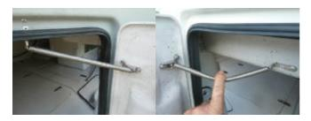
**D13.** These window covers slide into a sail track fitted above the window. It is supported by aluminium struts and rubber straps.
