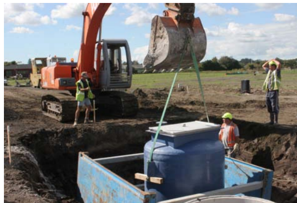
Photograph 8: Excavator installs pump station
