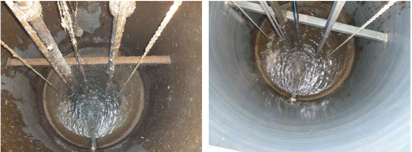
Photographs 5 & 6. Fibreglass pump station before and after 5 minutes cleaning with hose.
