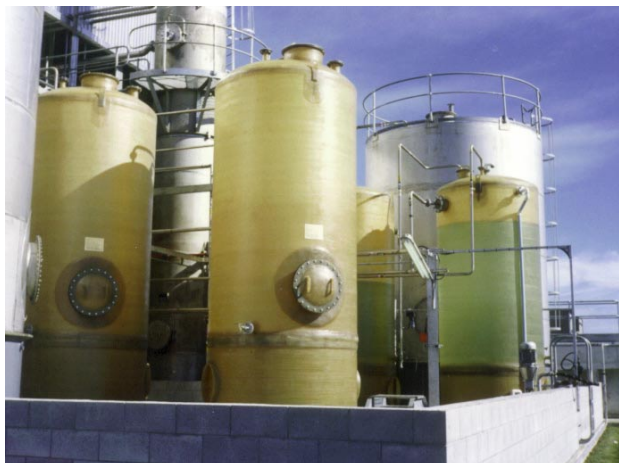
A series of fibreglass tanks at a chemical plant. Tanks with a natural translucent finish allow the liquid level within the tank to be observed from the outside.
