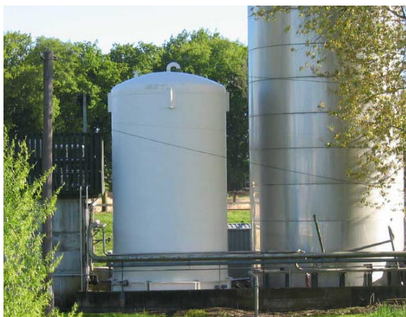
Fibreglass tank storing corrosive chemical located at dairy factory.
