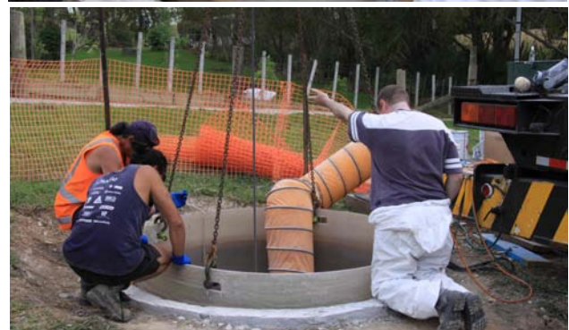
Lowering the FRP Liner into place ready to make off inlets and grout the annulus. Use safe practices at all times - H 2 S monitoring equipment, fresh air forced fed, and personal protective equipment.
