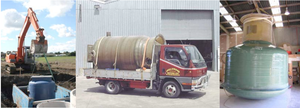
Fig 5: Fibreglass pumping stations prefabricated off site
