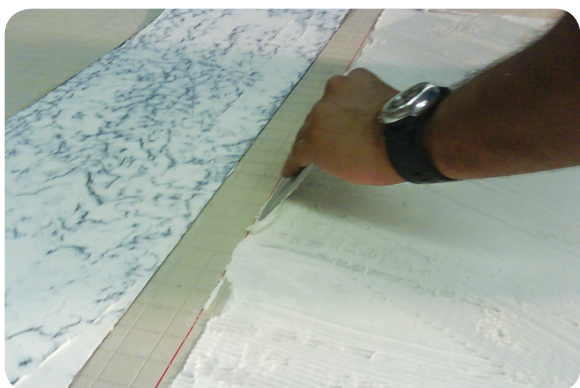
Back Fill and Trowel
