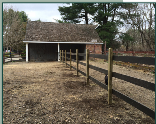
The new fence line is ready for horses
