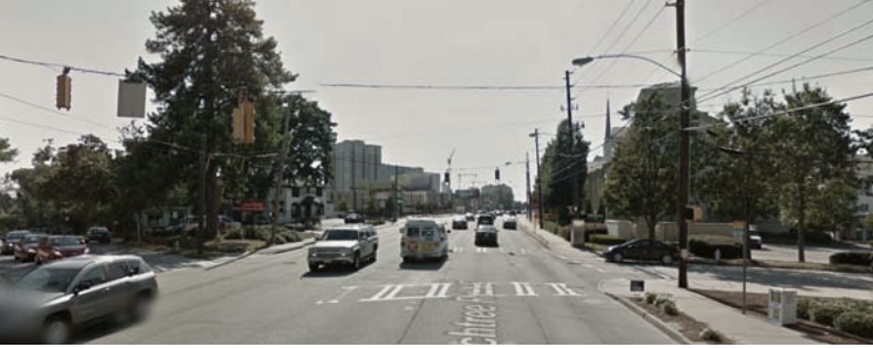
Existing 6-lane conditions
