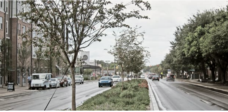
Planted center median with parallel parking.
