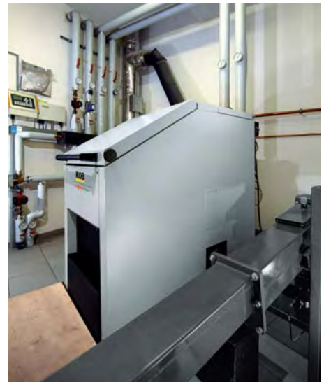
Pyromat DYN with spring core discharge
