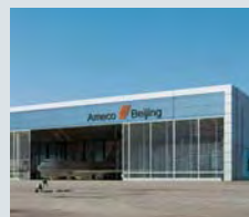
Ameco A380 Hangar Beijing, China
