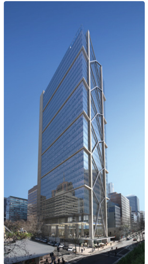
above left: Lauren L Stromberg, Analysis of cantilever cross-bracing, University of Illinois at Urbana-Champaign, Urbana, Illinois, 2012 above right: SOM, Office building, Sydney, Australia, 2012 In the diagram on the left, researchers at the University of Illinois, in collaboration with engineers at SOM, demonstrated that the optimal location for the intersection point of a cross-brace was not the midpoint, but instead a position somewhat above the midpoint, again confirming the relevance of the Michell frame. The rendering on the right shows the application of the optimal brace design on an office building.
