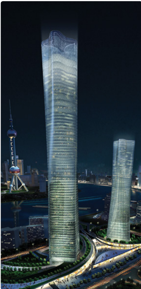
SOM, White Magnolia office tower, Shanghai, China, 2010 A gradient-based optimisation algorithm was used to identify the most efficient arrangement for a structural system for a pre-established complex building shape.
