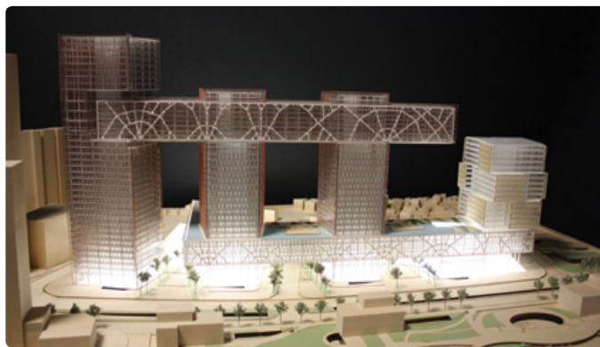
SOM, Commercial development project, Shanghai, China, 2011 A gradient-based optimisation algorithm revealed an irregular pattern for an optimal structural system for the bridge component of this project, which was incorporated as part of the architectural tectonics.
