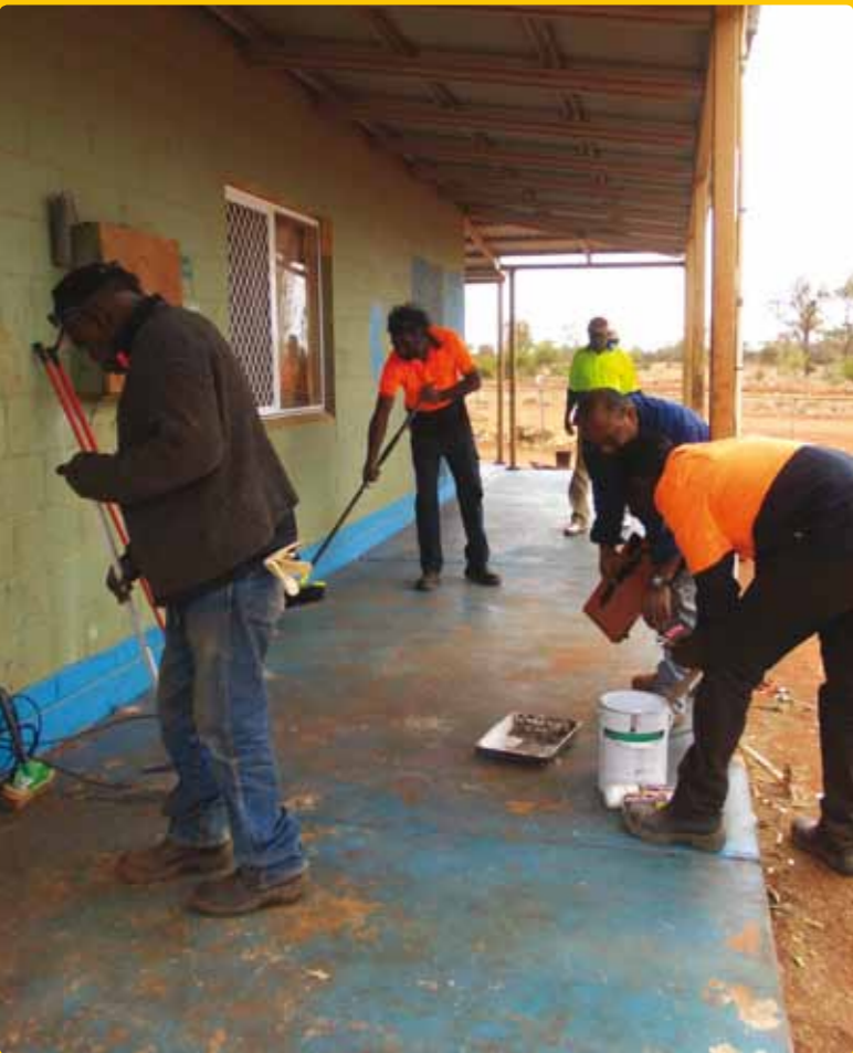
LEFT: The work crew clean a verandah in preparation for painting.
