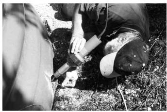
Some types of leaks can be repaired with a chemical sealant or plastic welding. Pictured above, a crack in a tank is being plastic welded with an appropriate plastic welding rod after first being stabilised.
