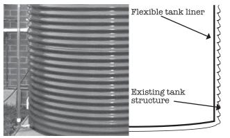
Flexible liners can be fitted to tanks to stop them leaking where they are still structurally sound. In other cases, a leak may be caused by the failure of a previously fitted liner to a non-water tight tank.
