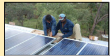
Mabunji staff installing system at Goolminy
