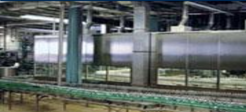
FrieslandCampina Domo, Manufacturing Expansion Delhi, NY
