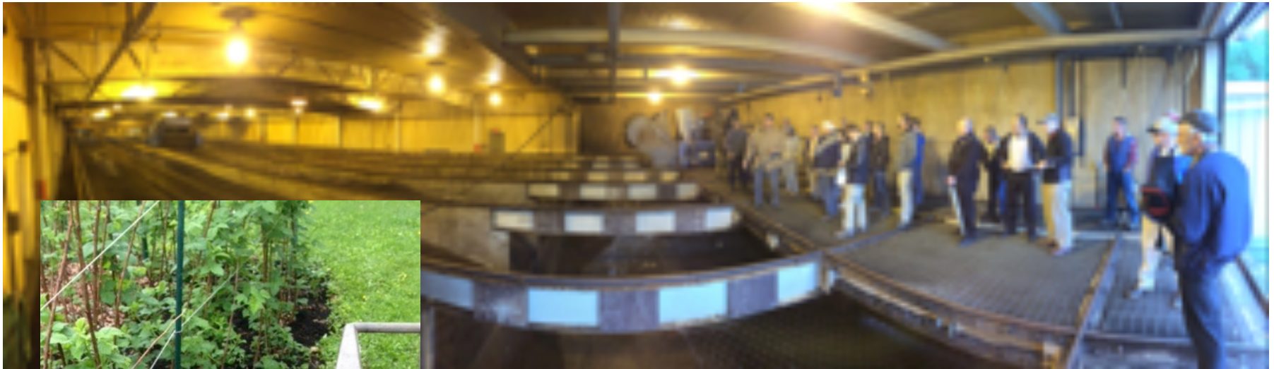
Lewiston-Auburn WPCA biosolids composting facility
