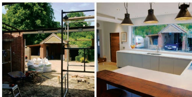
Garage conversion – before and after photos
