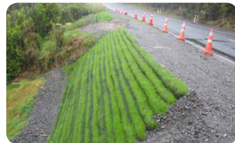
Plants are integral to Living Walls structural capabilities. Seeded grasses help provide initial stability until larger plants become established.
