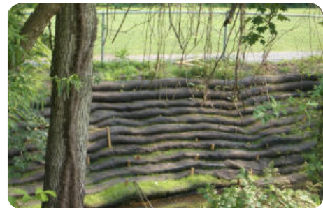
Living Walls are laid and staked to banks, or stacked and backfilled with soil.
