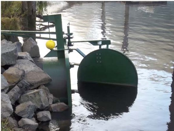
This NSG6ra tidegate is equipped with a coupling sleeve, an aluminum headwall assembly, an anti hammer device and a MTR unit.
