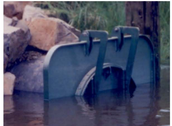
This is an NTG4oa tidegate before and after installation.
