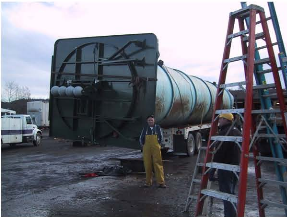
This is an NSG9ra tidegate before and after installation. Its auxiliary door is a mitigator type controlled aperture.
