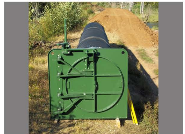
This is an NSG6ra tidegate before and after installation.
