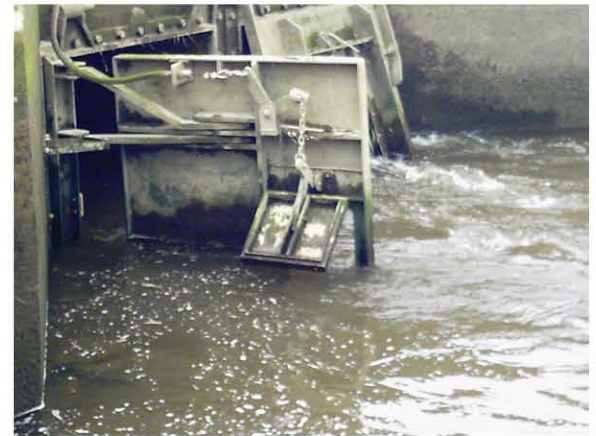
This NSRG5x6 tidegate is equipped with a auxiliary door which is controlled by an small MTR system.
