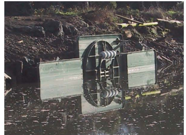
This is an NSG9ra tidegate before and after installation. Its auxiliary door is a mitigator type controlled aperture.
