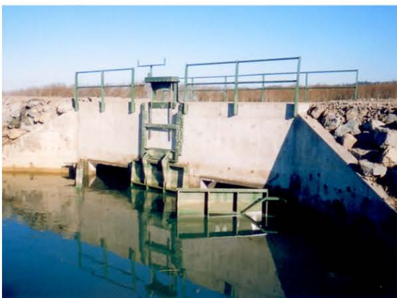
This NTRG 6x8 rc tidegate is fitted with a manual/curtain adjustment system to allow fish passage. Also shown are two NSRG 6x8 oc
