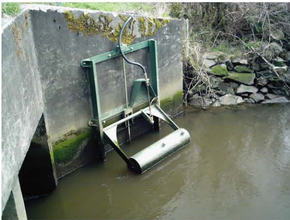
This NSRG5x6 tidegate is equipped with a auxiliary door which is controlled by an small MTR system.
