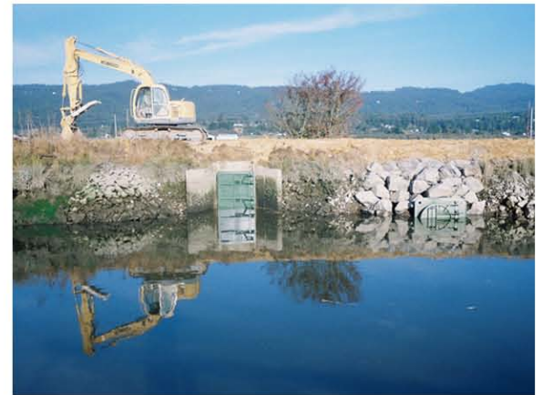
This is an NSRG 5x6 tidegate installed in Arcata, CA. The NSRG 5x6 is mounted to the concrete.
