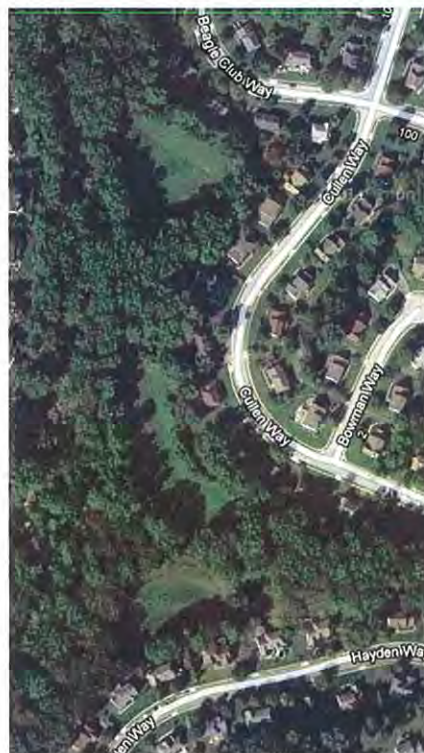
The three basins at the Hunt at Louviers were each apparently designed as dry basins. Though fairly typical in the day, this type of facility may mitigate storm flows but does little for stormwater quality.
