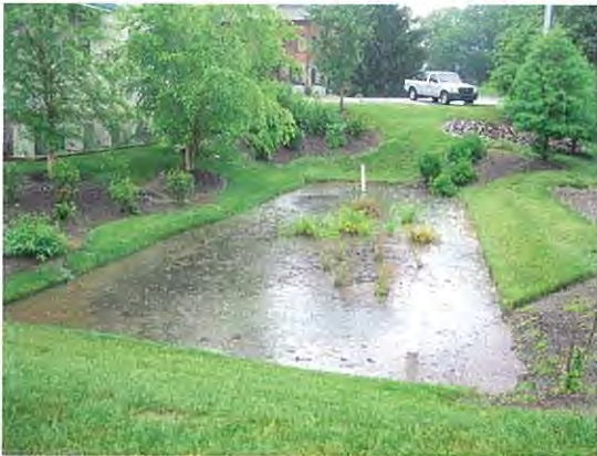
Duffield's headquarters, just 10 minutes from Newark, includes innovative bioretention design for stormwater management.
