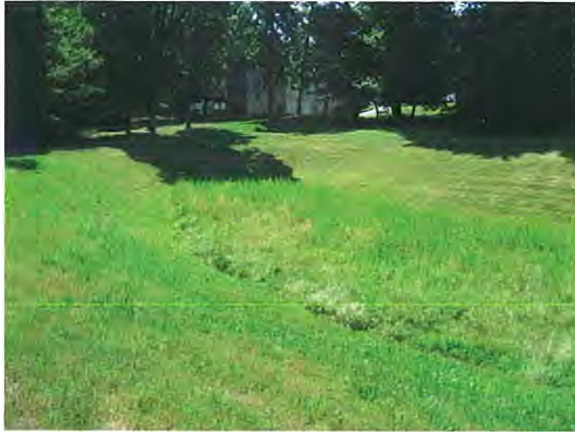
The Hunt at Louviers Detention Basin No. 2 (middle basin) is currently dry throughout most of the year and drains quickly after storm events.
