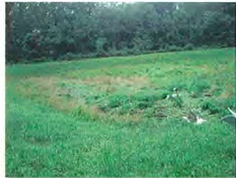
Basin No. 1 (northernmost) as viewed from above the inlet pipe. On the wet day this basin was observed, only the area immediately in front of the inlet structure remained wet. Re-grading for native plant communities will allow nutrient uptake and infiltration for the entire basin bottom.
