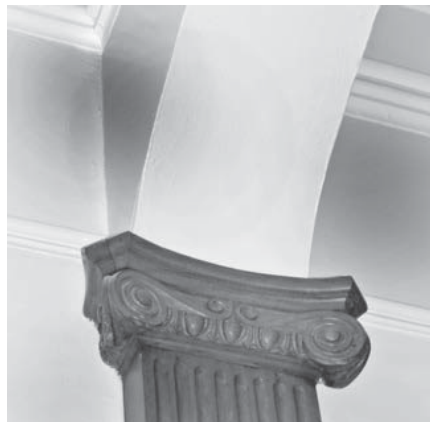
Retaining decorative plaster, moldings, and details saves original materials, embodied energy, and costs. Often the craftsmanship represented by finishing details is costly, if not impossible, to replicate.
