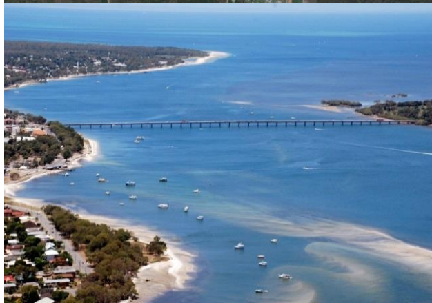
Bribie Island bridge
