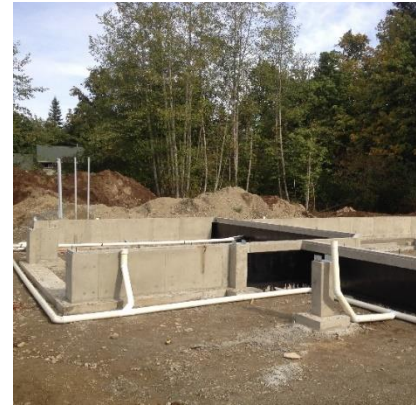
Figure 1 - Foundation poured and set
