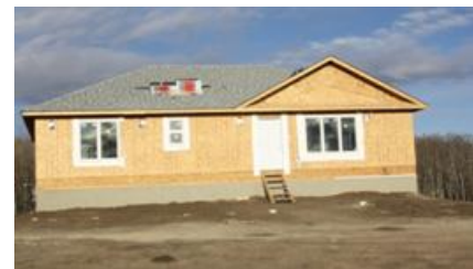
Figure 7 - A First Nations home nears completion
