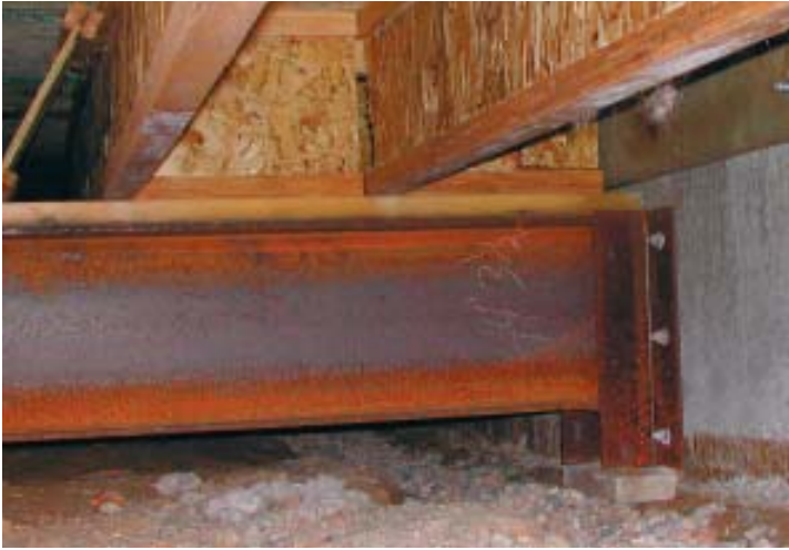
Figure 8. Steel saddles, expansion-bolted to the foundation walls, support the ends of the central girder in the crawlspace (above). The ends of the I-joists rest in joist hangers fastened to pressure-treated ledgers (right).
