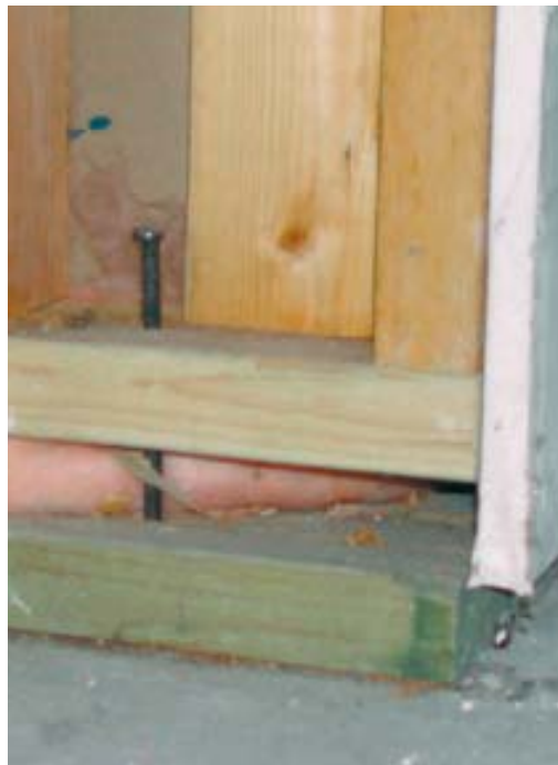
Figure 7. Where basement slabs are used in expansive-soil areas, a “floating wall” detail is used to prevent possible heaving from displacing the floor above. A pressure-treated sill plate is powder-fastened to the slab. The partition wall, which is constructed 2 inches shorter than the height of the basement, is temporarily positioned with wedges between the treated sill plate and the bottom plate of the wall. After the top plate has been nailed to the overhead joists, a 60d spike is driven into a slightly undersized predrilled hole in the bottom plate of the partition and into the treated sill plate. The baseboard is nailed to the sill plate but not the wall itself, so any movement of the slab will not distort the partition.
