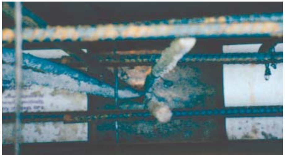
Figure 6. In a top view into the forms just before the concrete pour, the void forms are visible at either side of the caisson at center (above). The vertical strands of rebar extending from the caisson will anchor the foundation wall to the caisson, which will bear the structure’s weight. After the forms have been stripped, the edges of the void forms are visible at the base of the wall, except where interrupted by caissons (left).
