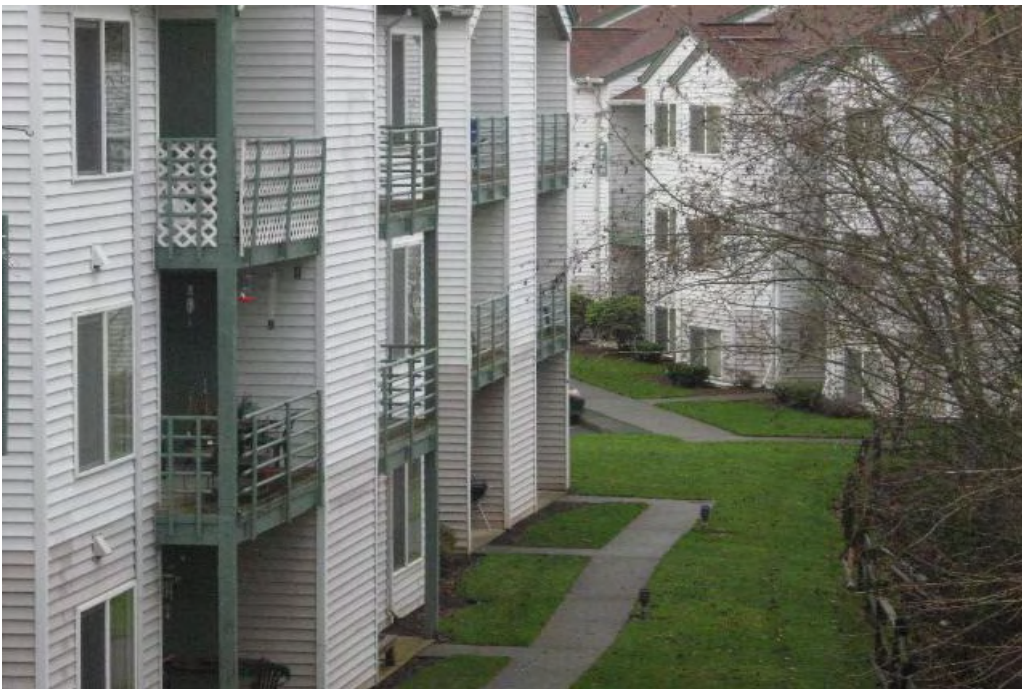
SM 01.056 Unit #29; Back elevation; Looking east, typical building.
