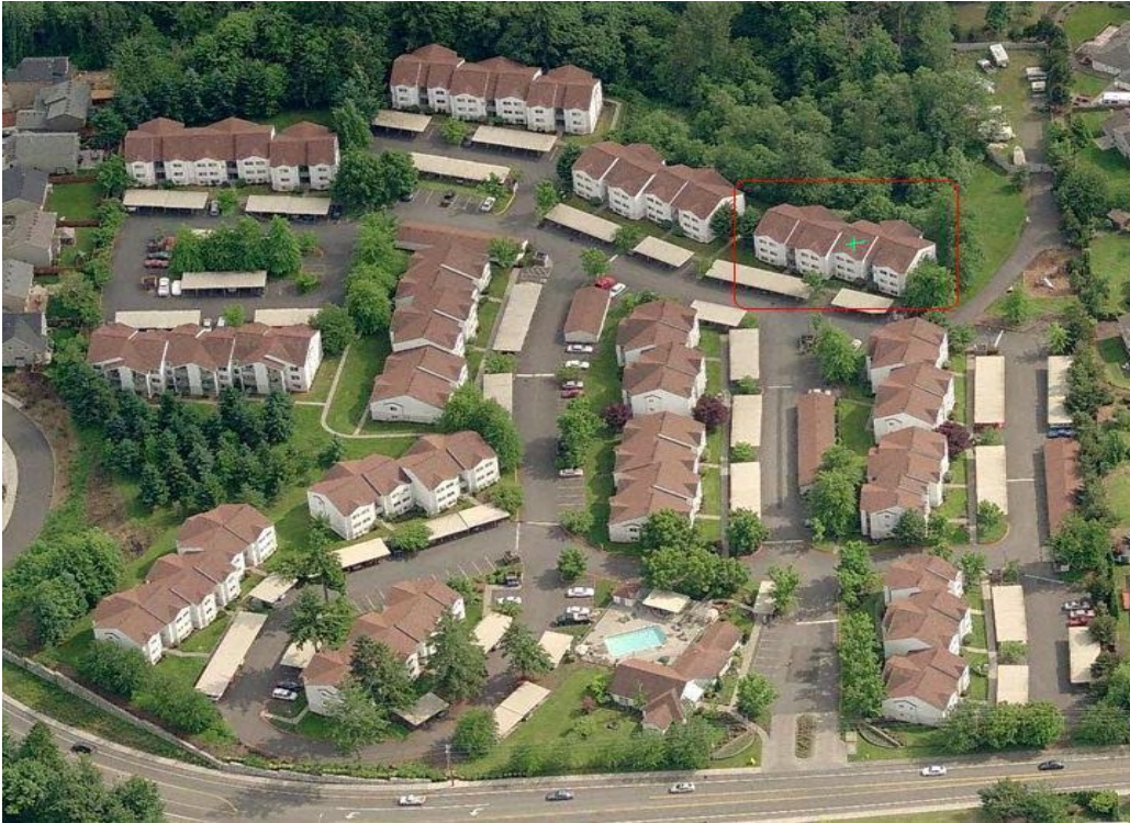
local.live.com – Aerial Image (Building C is outlined in red)
