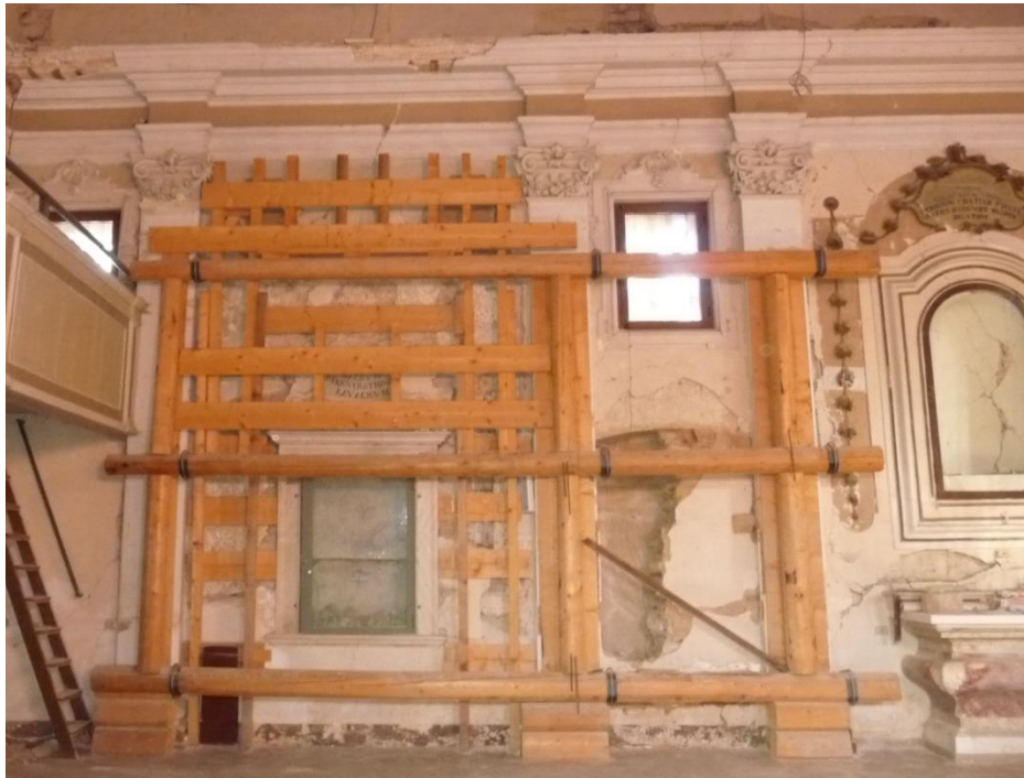
LEFT LONGITUDINAL WALL – PRESENCE OF OPENINGS AND NICHES
