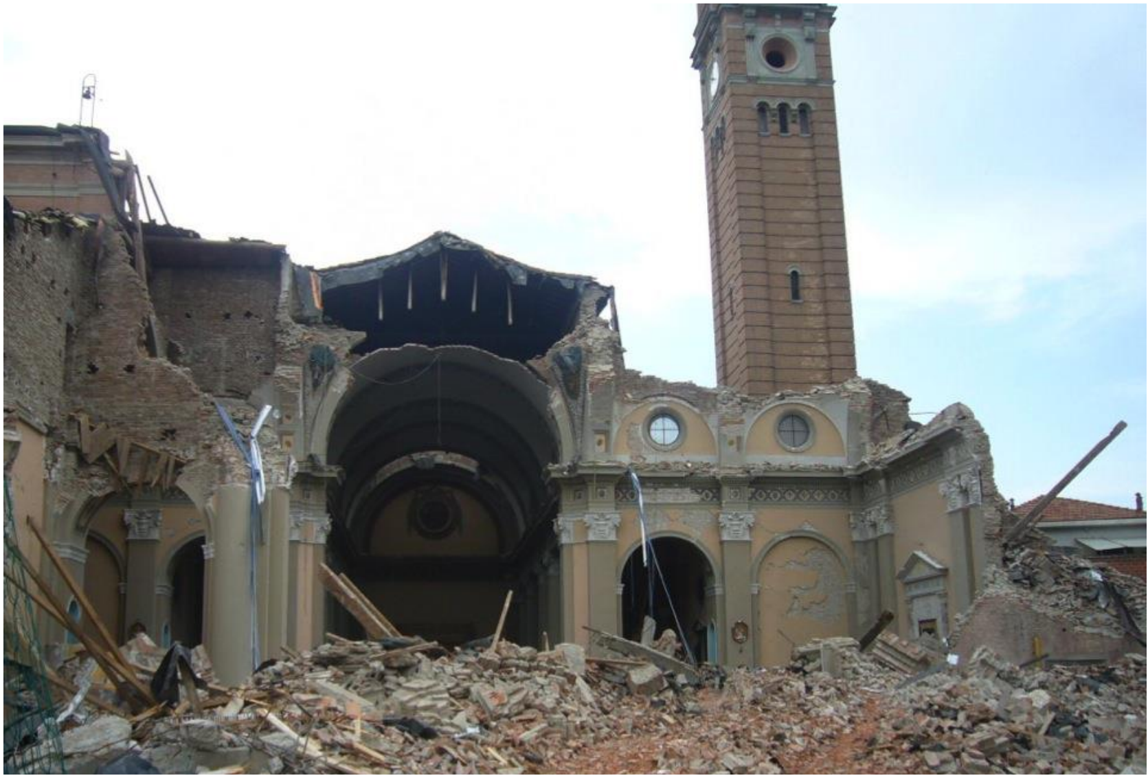
Church and bell tower in Mirabello: isolated bell tower
