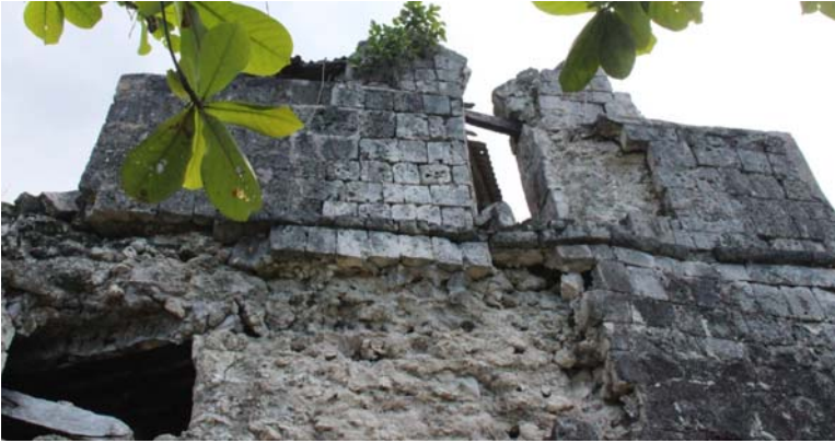
No connection of the external leave to the inner core
