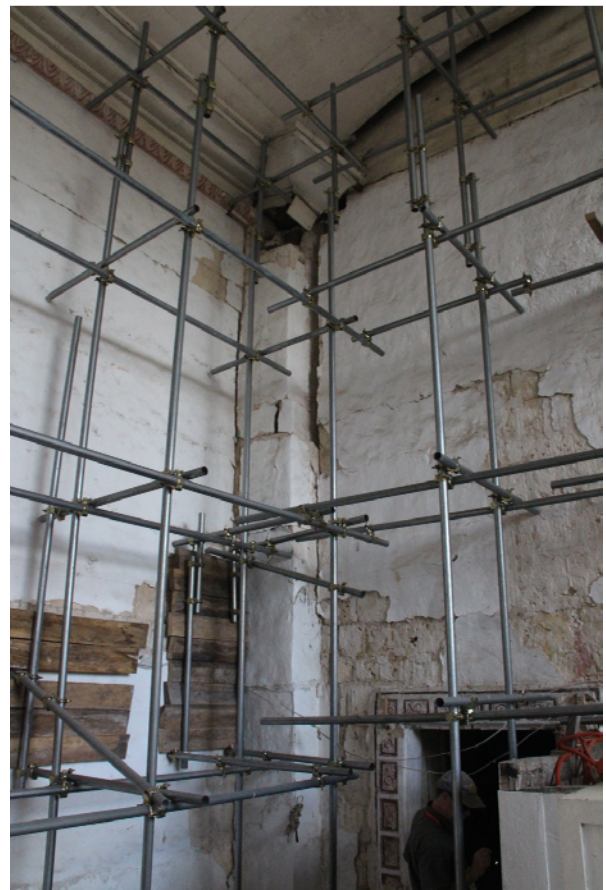
Lack of connection between transverse walls
