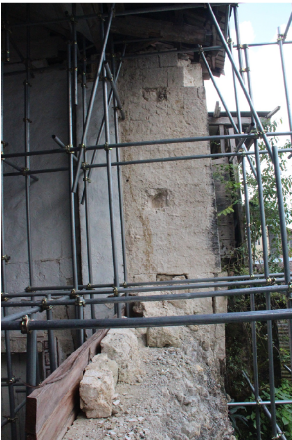
Lack of connection between transverse walls
