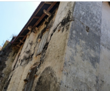
Extend to the corner. Reinforcement
