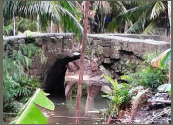
BRIDGE, DIMIAO, BOHOL
