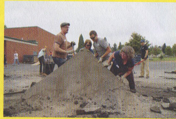
Depave. Depavers at Lewis Elementary School, Portland, Oregon. 2011
