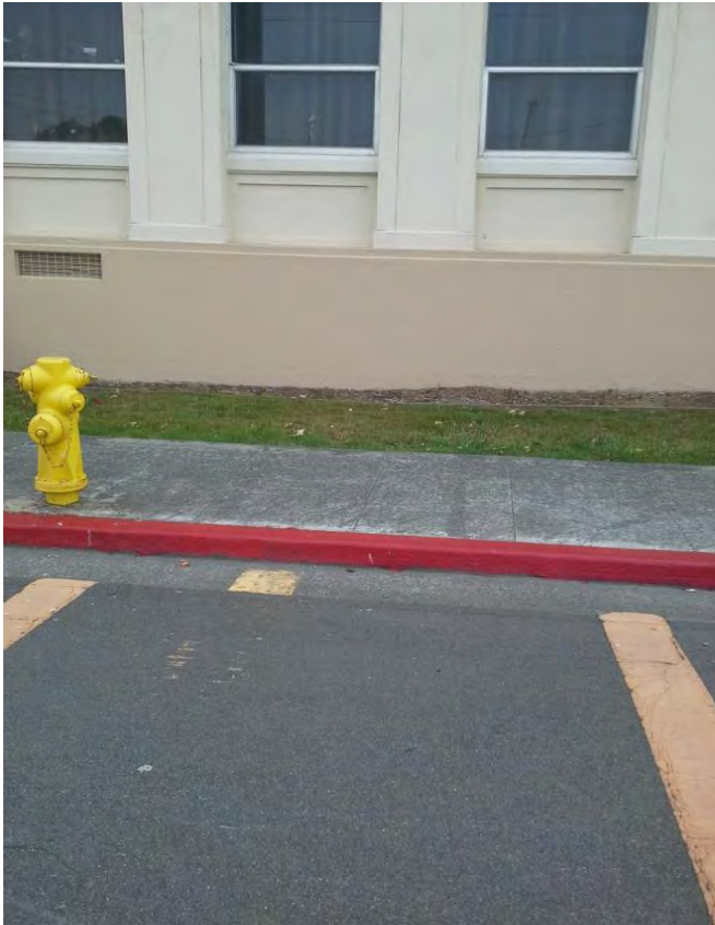
Crosswalk lacks curb ramp
