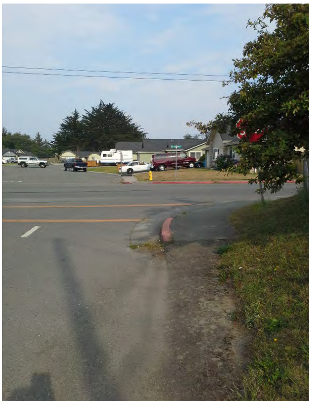
Unfinished sidewalk-Not compliant with ADA and poses a tripping hazard.
