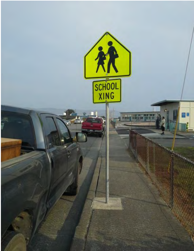
Signage is important to warn drivers, but the location of this sign makes the sidewalk too narrow for ADA compliance
