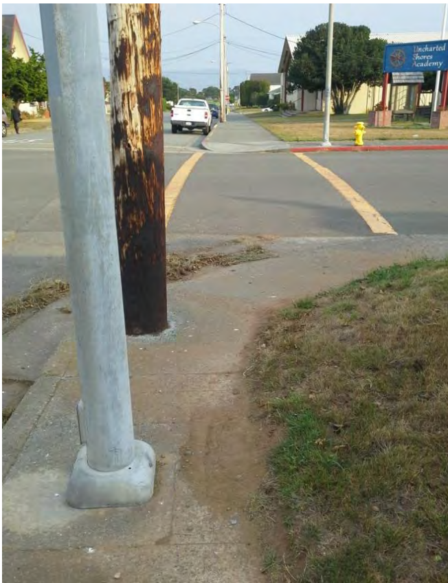
Sidewalk blocked by utility pole and light standard
