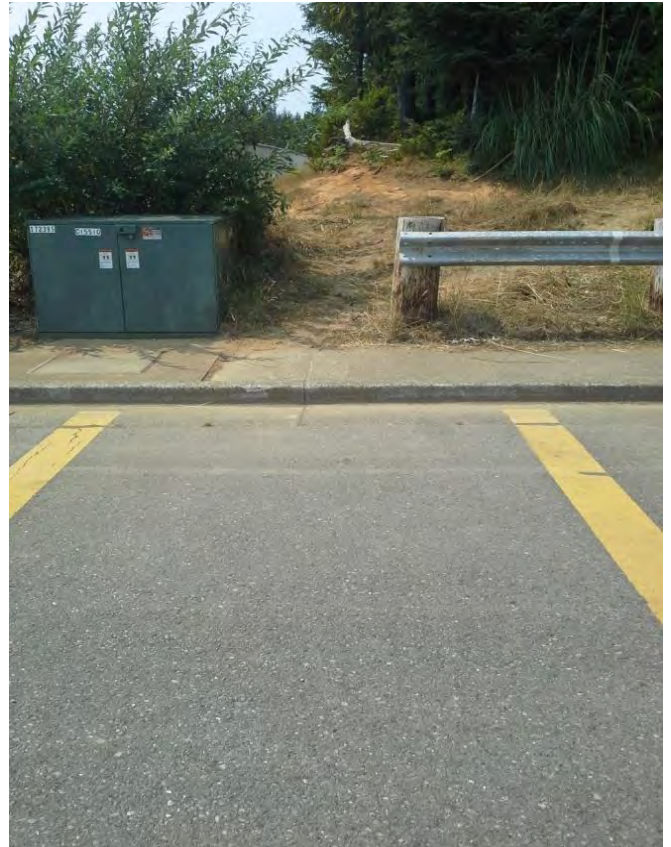
Crosswalk doesn't have an ADA accessible ramp
