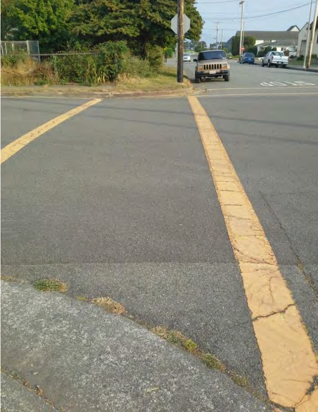
Crosswalks lack curb ramps and sidewalks on opposite side
