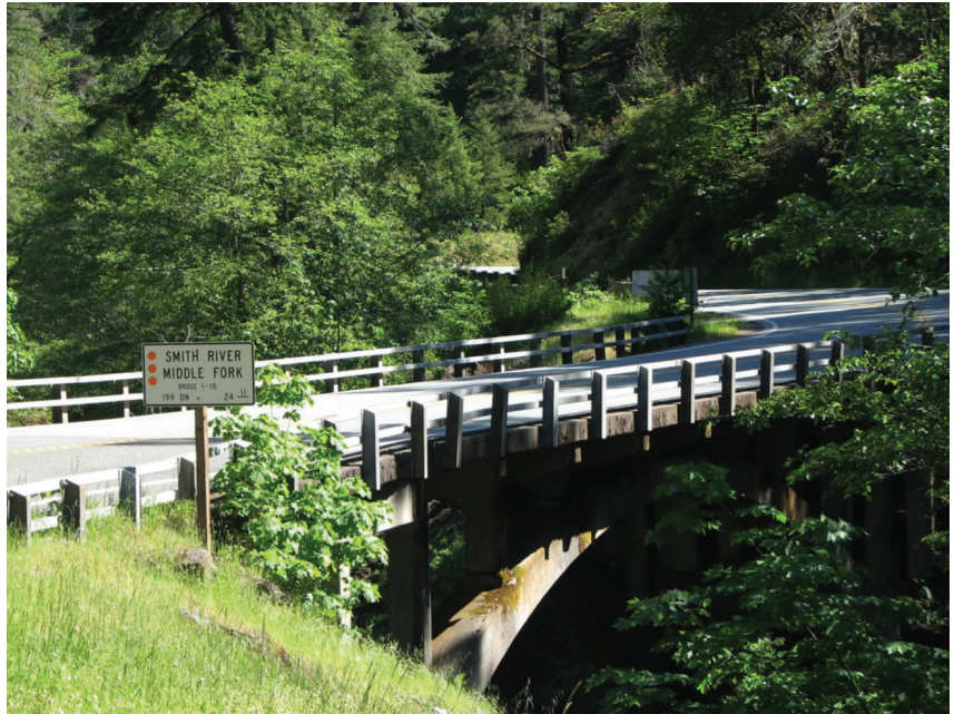
Existing Curves on the Middle Fork Smith River Bridge
