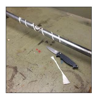
Wrap diagonally with overlapping turns.
