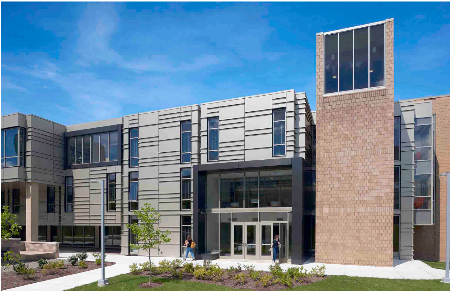
Binghamton University, Science IV – A southside view of the building shows the new main entrance, new metal cladding, third-floor infill, and the existing tall masonry stairwell. (Photo Credit: David Lamb Photography)
