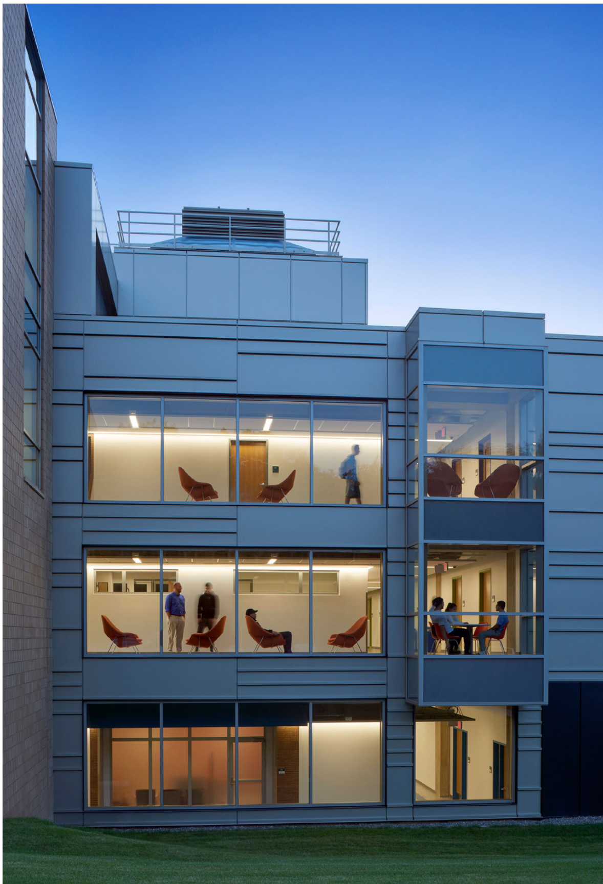
Binghamton University, Science IV – A westside view of the building shows a portion of the new metal cladding (added to the exterior), new windows, and a glimpse of new interior collaboration spaces. (Photo Credit: David Lamb Photography)
