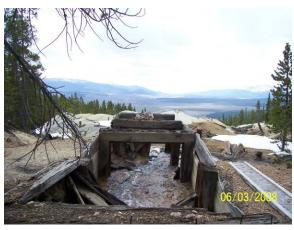
Acid mine drainage from the collapsed Tiger Tunnel runs across the large mine waste pile.
