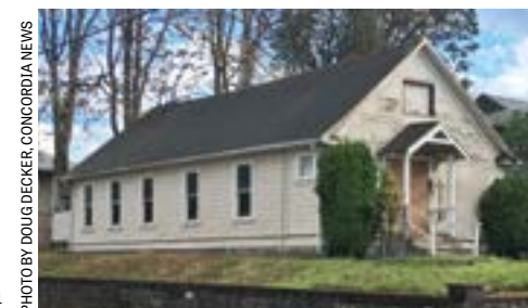
This is the building today. Developers have been eyeing the lot as a tear-down. The Alberta Shul Coalition has secured an agreement with the current building owner and is raising funds to purchase and restore the 117-year-old building.
