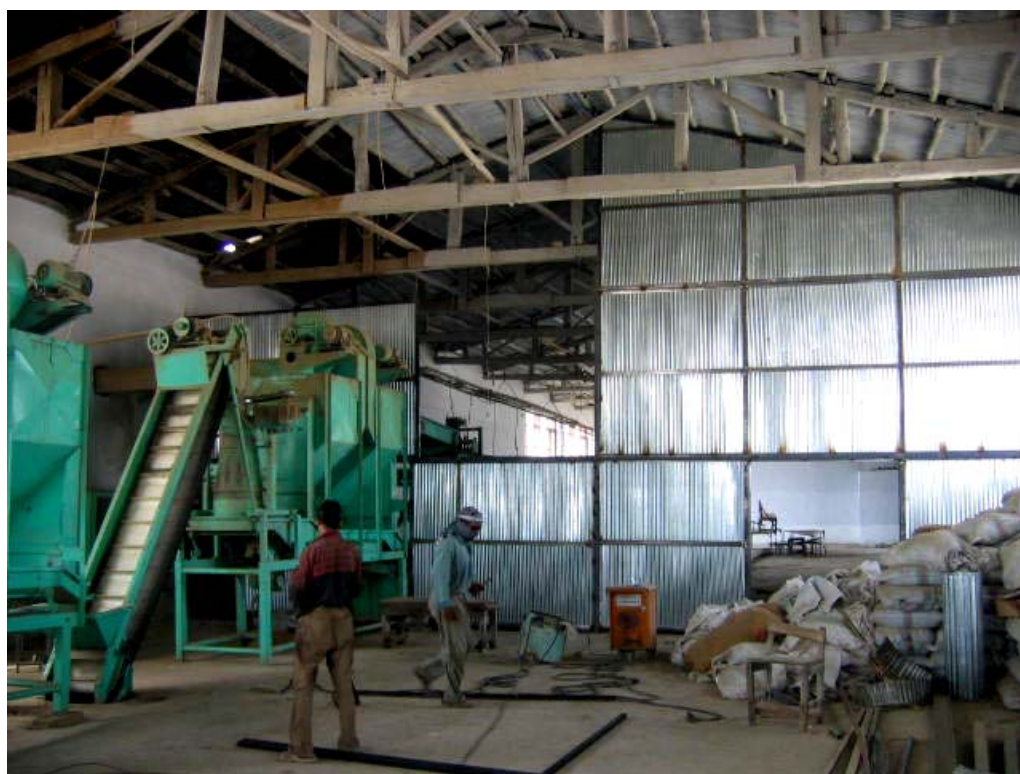
Construction of curtain wall inside Rahmat Raisin Plant to seal-off dusty area from clean area of the plant, August 2005.
