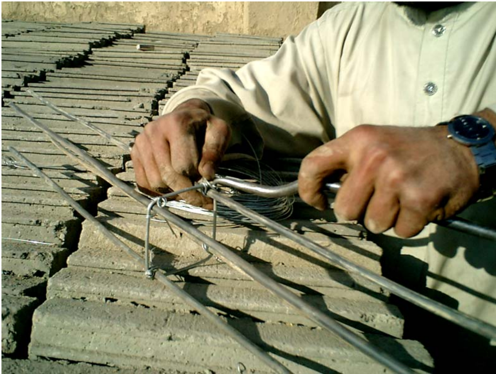
Detail of iron used inside concrete trellis posts, February 2006.
