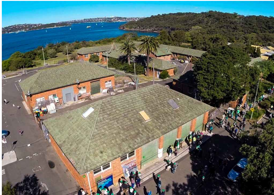
VIEW 02_BIRD'S EYE VIEW OF EXISTING BUILDINGS
