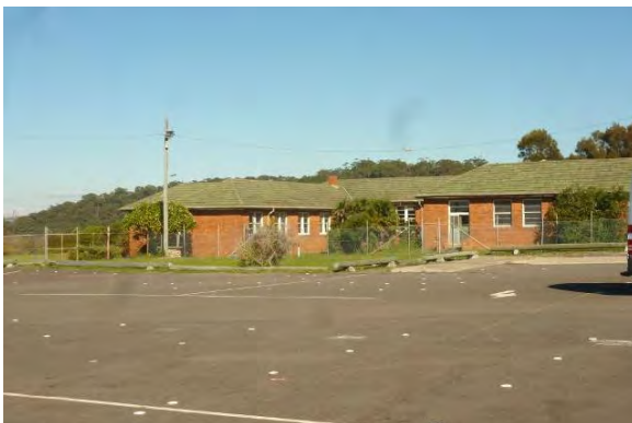
Figure 14 Looking south west towards Building 3 from the adjacent public car park.
