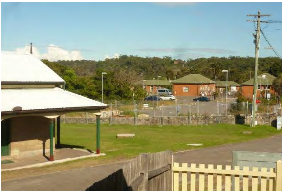
Figure 20 Second view looking south west towards Ten Terminal buildings.
