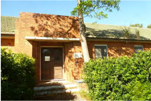
Figure 7 The main entry feature in the northern façade of Building 1.
