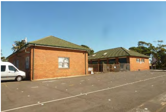
Figure 8 Building 6, on the left, will be demolished and replaced with a new two storey building that then links with Building 7, on the right.
