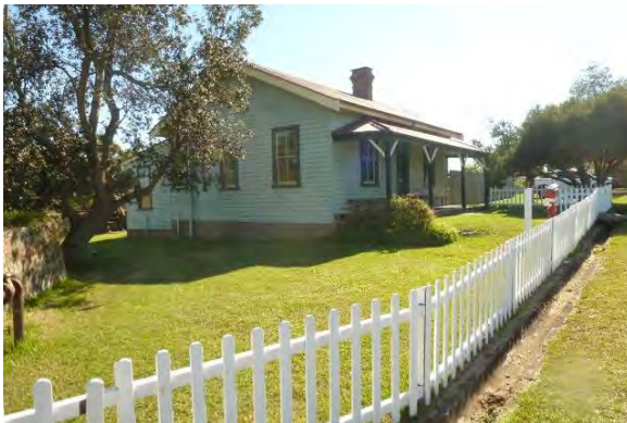
Figure 17 Timber cottage is located to the immediate north of the NPWS building
