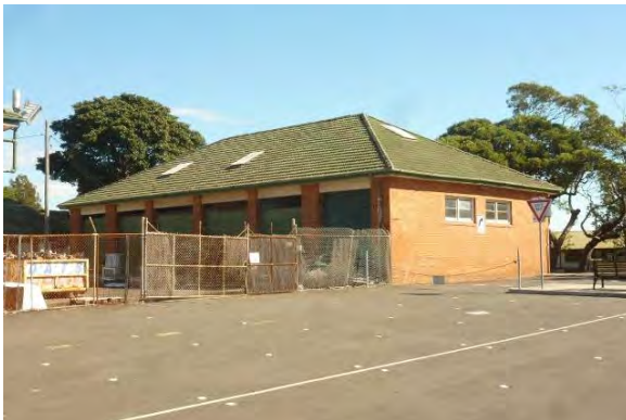
Figure 9 Building 7 is located right on the Middle Head Road frontage.
