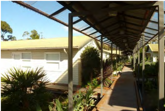
Figure 25 A covered walkway has been introduced to create a new internal pedestrian circulation spine through the complex.
