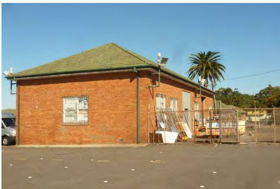
Figure 10 Building 6 will be demolished and replaced with the southern extension of the large two storey building
