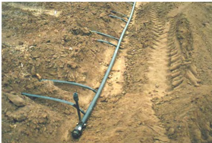
Flushing Manifold prior to burial.
